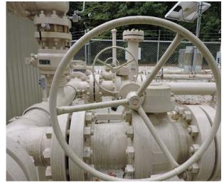
pressure when gas is moving on the "downstream" side of a pipeline. Regulators work in conjunction with reliefs to ensure that pipeline pressures remain within the design parameters. If a regulator fails, a back-up regulator, or relief, will activate to control the pipeline pressure.
