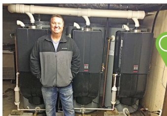
Captain Steve's Installation of three Rinnai Demand-Duo Water Heaters
