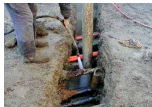
A communications contracting company struck a 2-inch gas line with an underground boring machine resulting in an explosion at a Kansas City restaurant.
